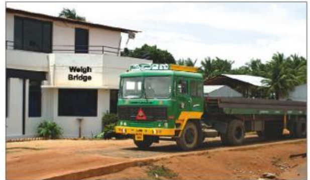
60 MT Weigh Bridge
